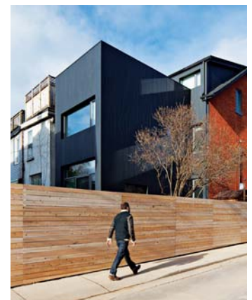
↓ The back of the house is clad in vertical strips of black-stained cedar, while the front remains typically Victorian. The fence is made of raw cedar.
