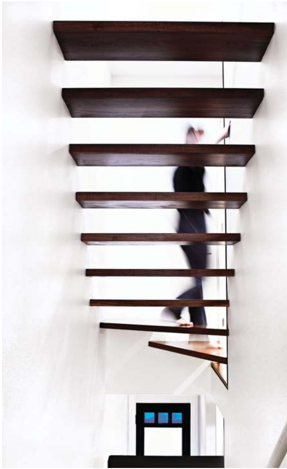
↑↗ Floating stair treads allow outdoor light to filter through the house, from the top floor down. Dubbeldam saved valuable centimetres in the stairwell by inseting the handrail right into the wall.
